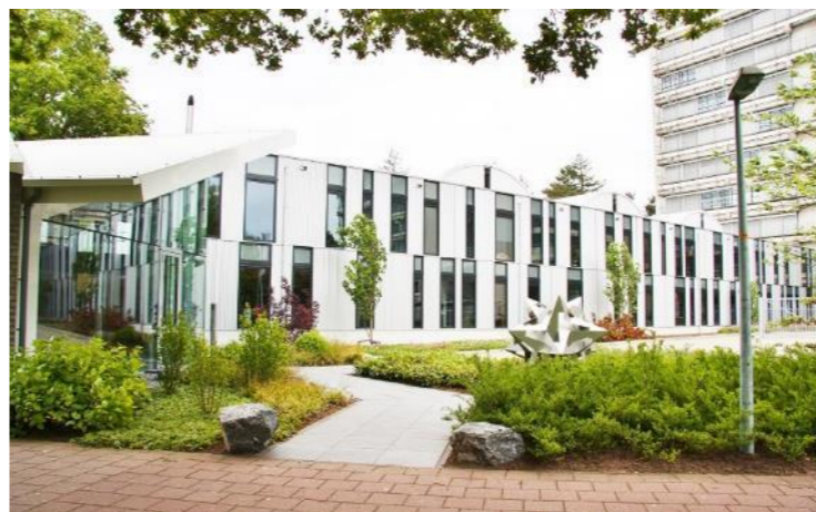
High Tech Factory, PHIX assembling & packaging Fab
